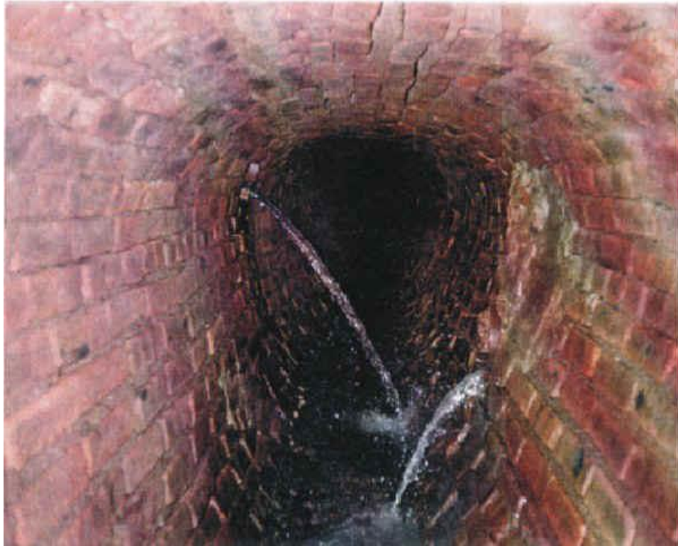
Horseshoe-shaped brick sewer under Mulberry Street near Lafayette Street built ca. 1870. (Photograph by Specialty Sewer Services, Inc.)
