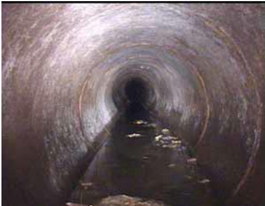
A clean sewer, without grease or oil build up, allows appropriate flow downstream.
