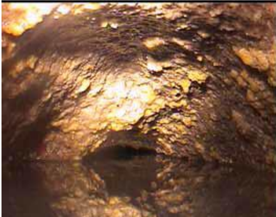
A dirty sewer, with significant grease and oil build up, hinders wastewater flow.
