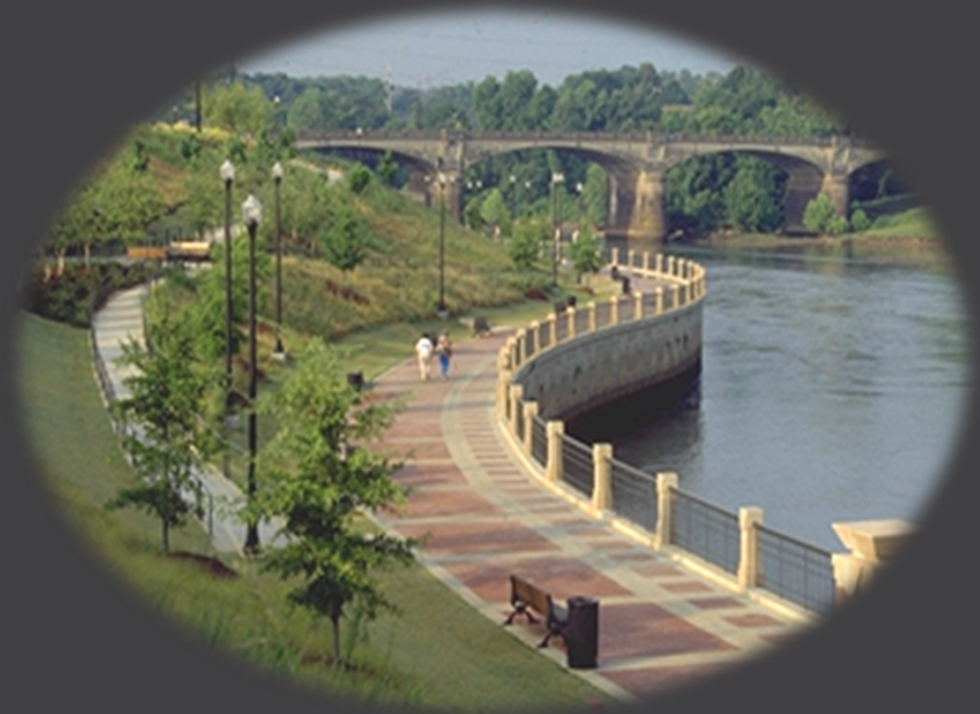
Walk/Bike Path Constructed over CSO storage/Conveyance Pipe
