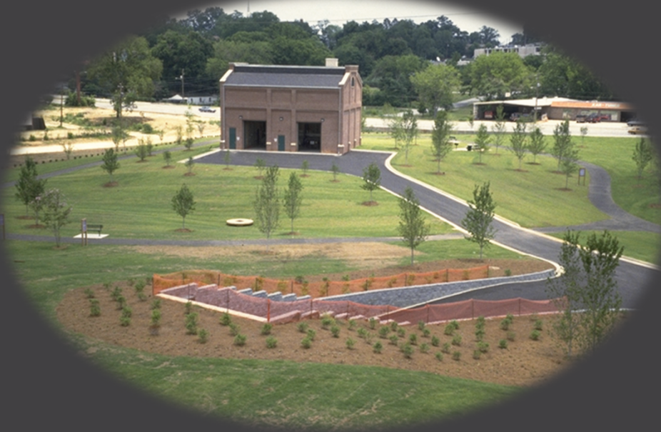
Park Constructed over CSO Vortex Facilities
